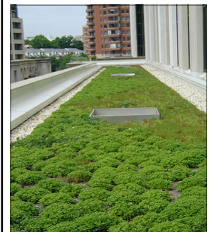
The vegetated "green roof" on the Arlington County Government Center
